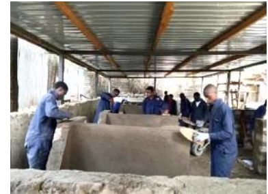
Wall finishing by plastering
