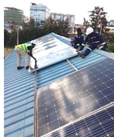
Installation of the solar panels
