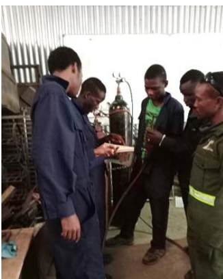
Students constructing a manhole chamber.
