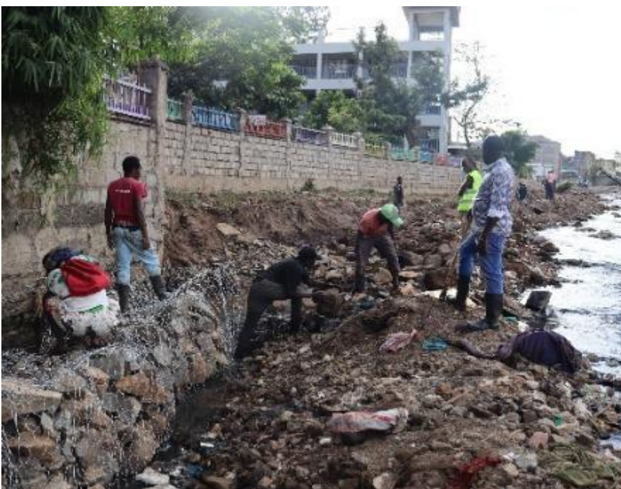
Initial stage on the gabions at Songa – Ngong River
