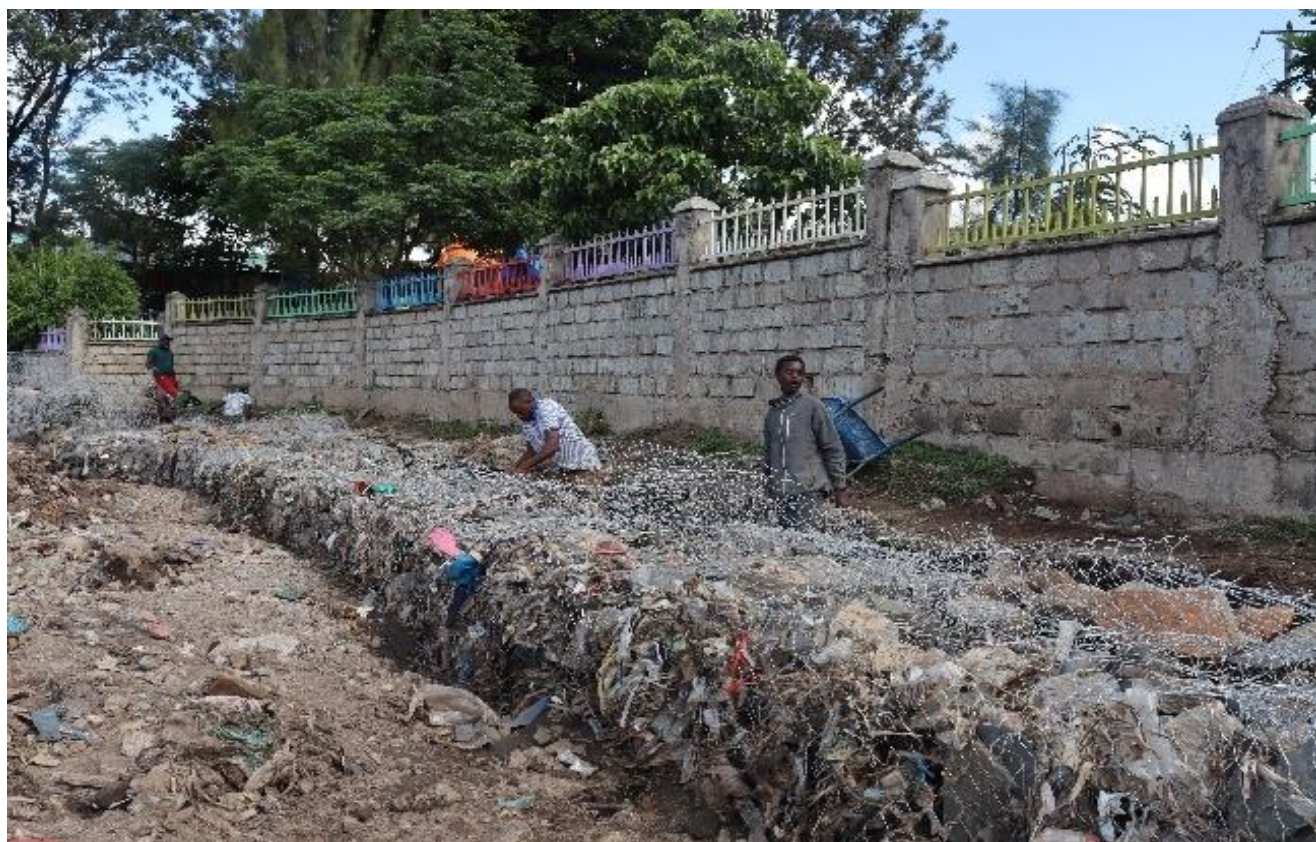
Gabion construction in the foreground and the wall in the background
