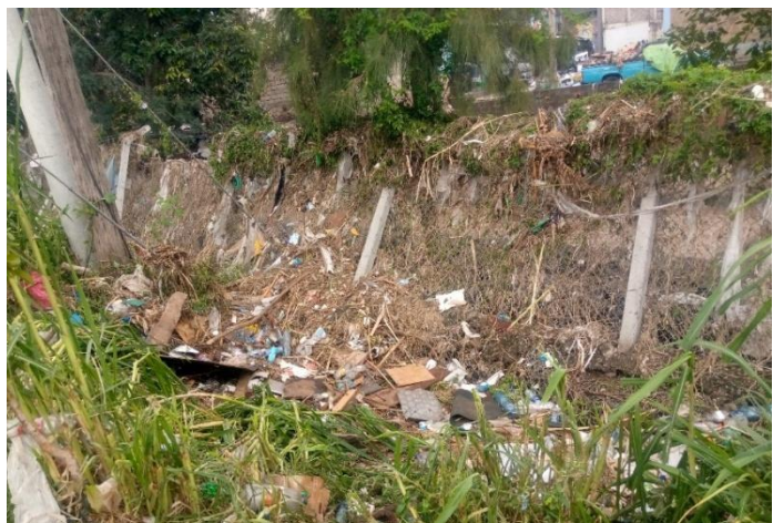
Large sections of soil were washed away
