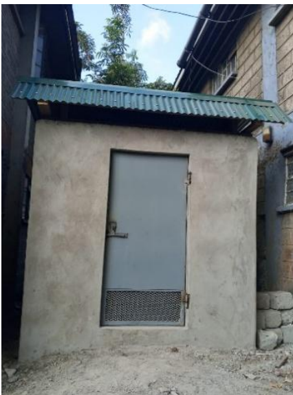
Generator storage room
