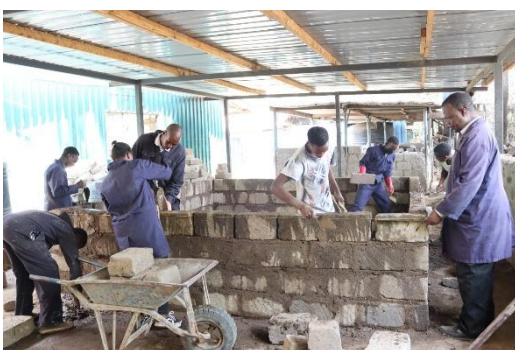
Plumbing and Masonry
