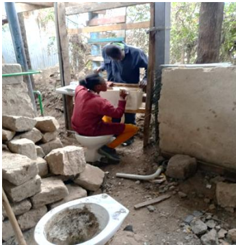
workshop repair, water linkage, and sink installation.
