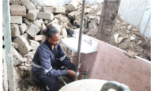
Installation of a washing hand basin
