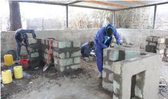
Masonry joining of blocks & plastering
