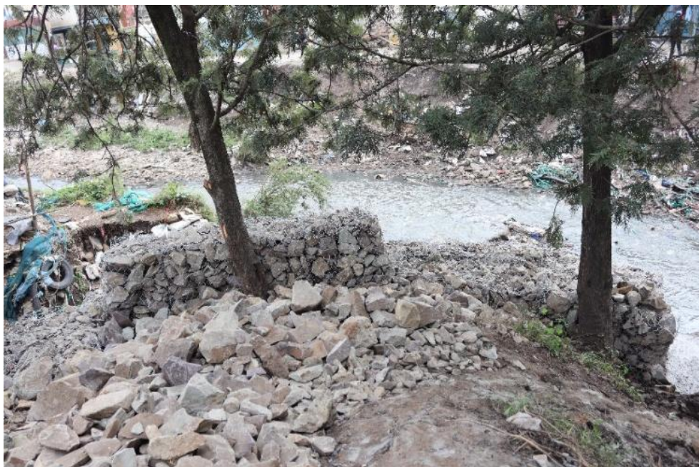
Continuation of gabion construction
