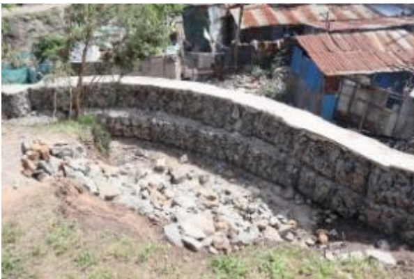
Gabion retaining wall construction along the river parallel to St Bakhita Primary School
