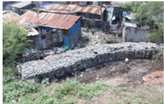
Gabion retaining wall construction along the river parallel to St Bakhita Primary School
