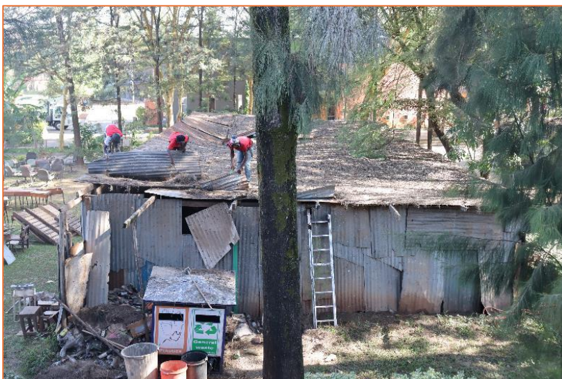
Last mabati structure at Head Office
