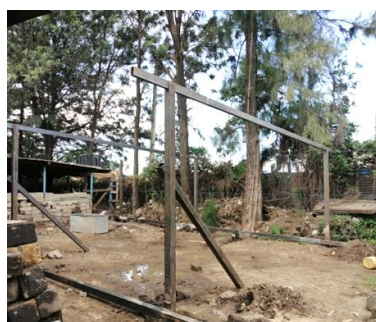
Welding of the roof panels and the erection of the pillars
