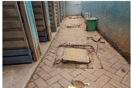
Repair of steel doors and sewer line.
