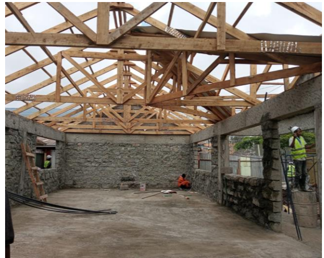
Roof frames in place
