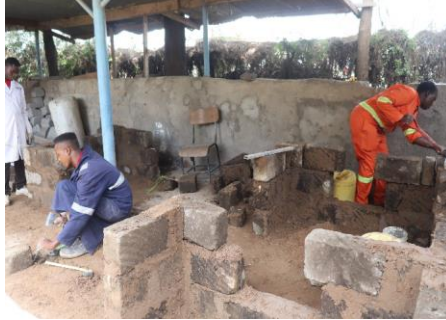
Masonry and Plumbing
