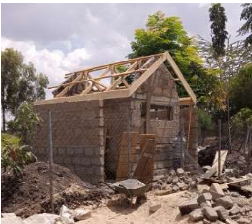
Construction at St Elizabeth and Sancta Maria Kayaaba
