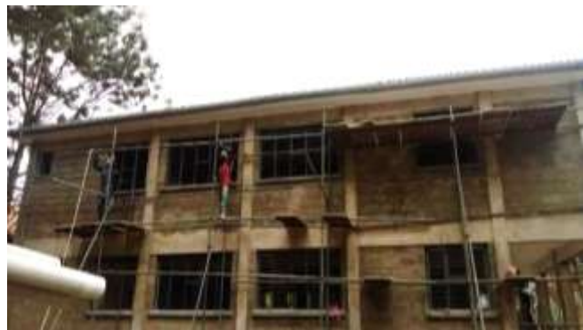
Fixing the gutters
