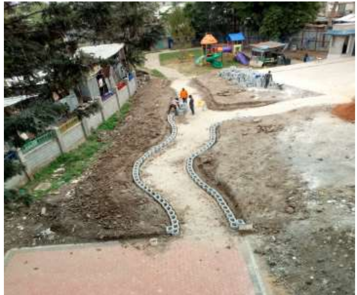
Aerial view of the pathways
