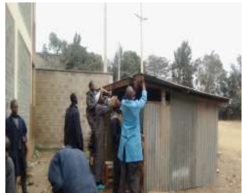
Constructing the dog kennel
