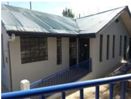
Renovation of the existing building
