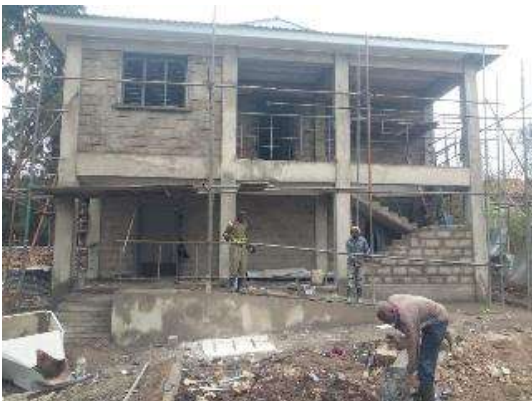
Fabricating and fixing the balustrades and handrails.
