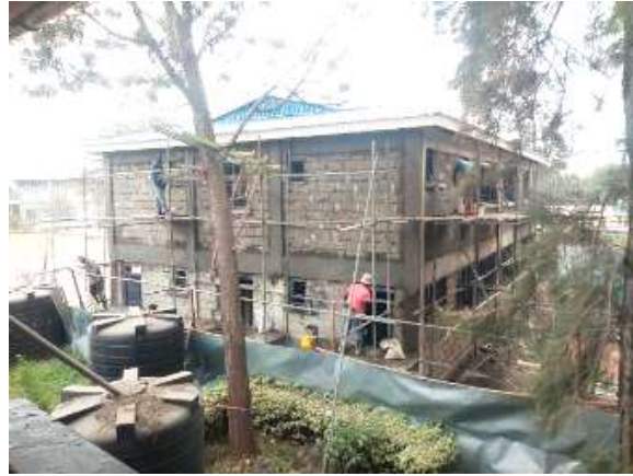
Columns and beams plastering
