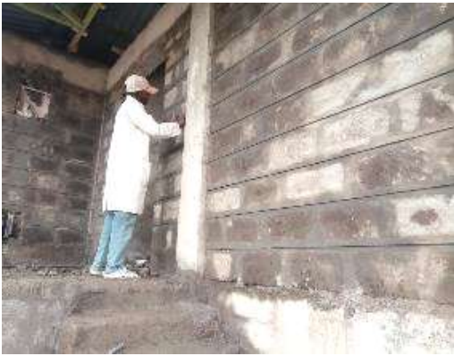
External wall finished (Keying).
