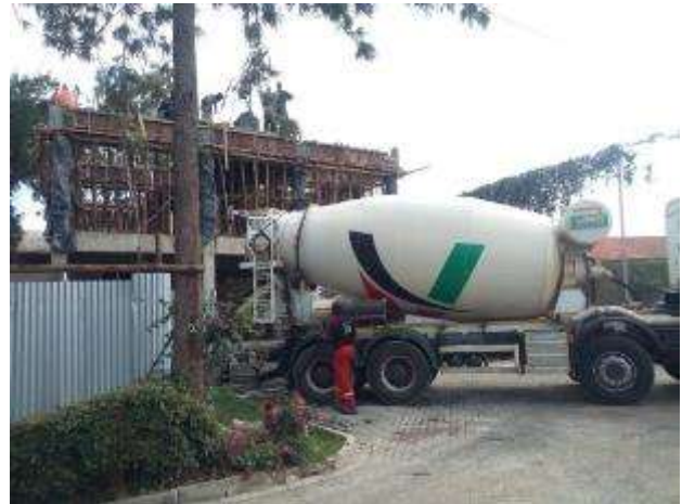
The first floor ring beam concreting
