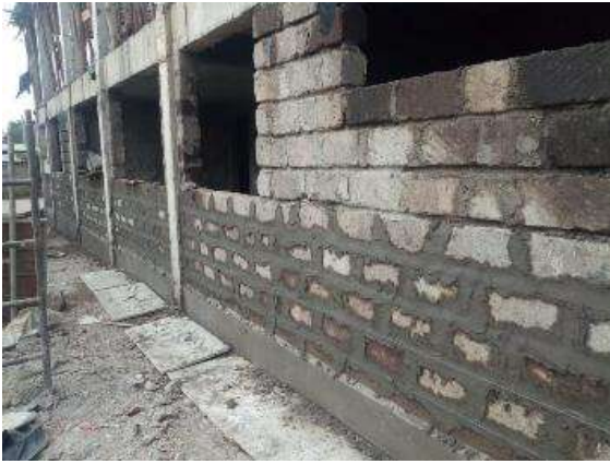
External column plastering / finishing
