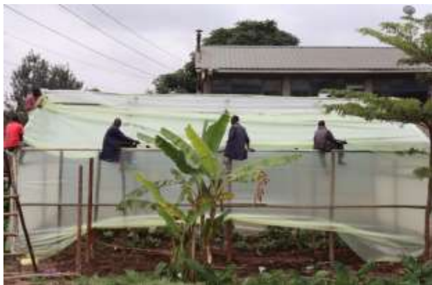
Carpentry students construct the donated greenhouse
