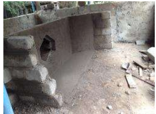
Walls constructed with finishes of keys
