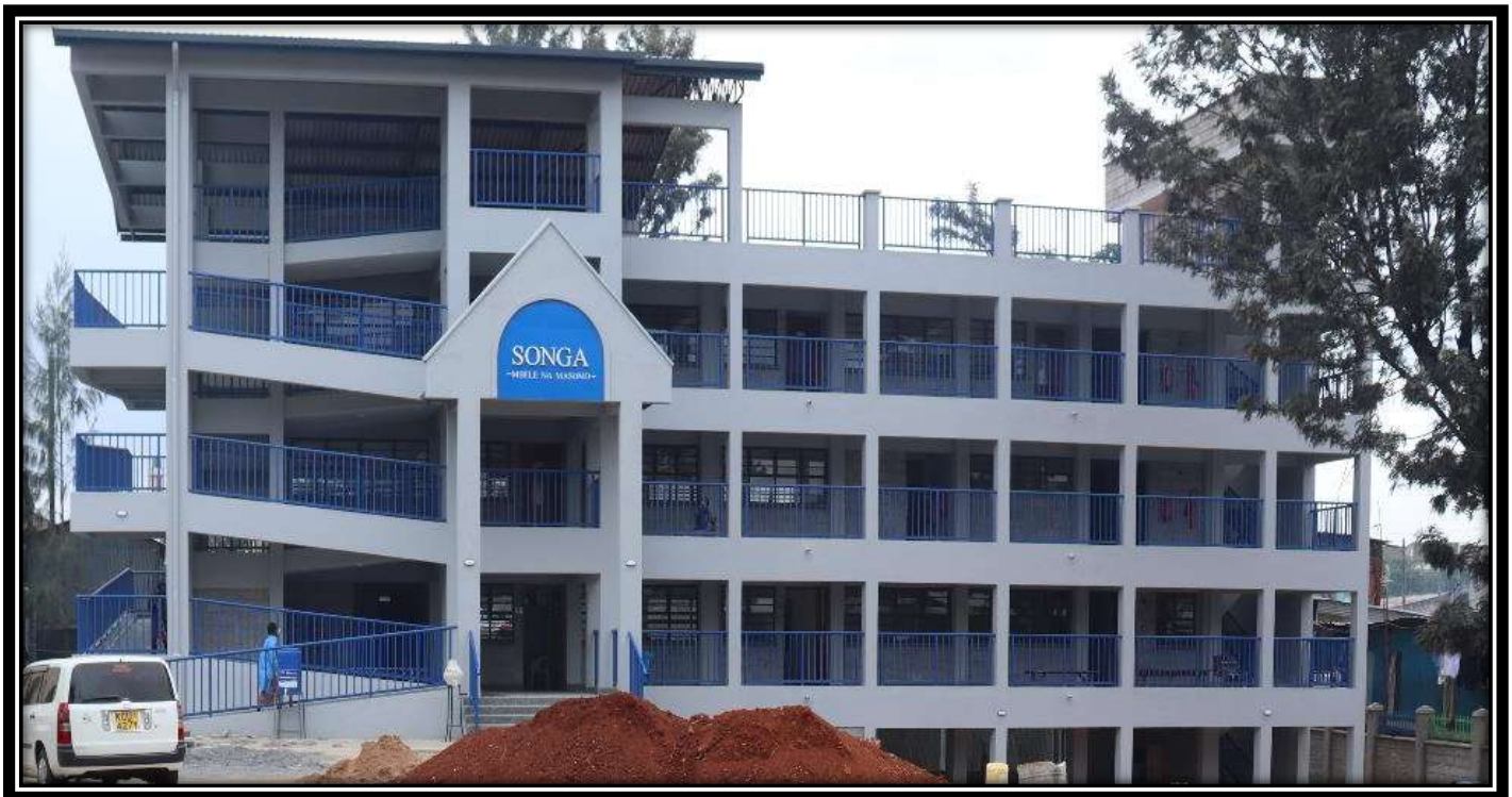
Multi-storey Facility – Sponsored by Kenyan Child Foundation Architect: Malinson Koech (Lins Consult) Contractor: Anshi Builders Ltd – Mr Vinod
