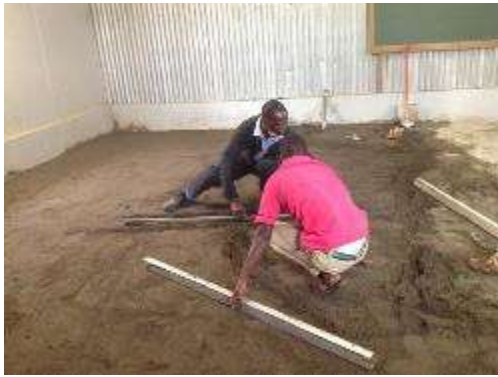
Catering classroom floor taking shape
