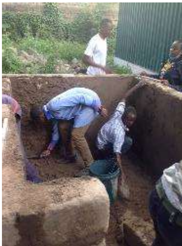
Plastering the wall
