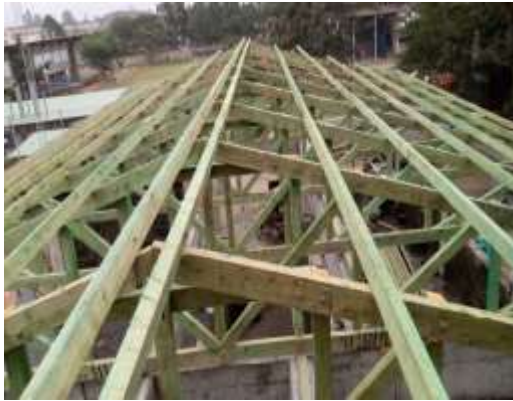
Roof structure showing set trusses and purlins
