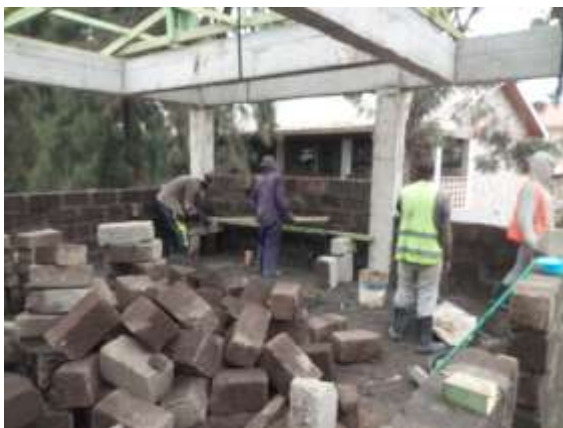
First floor walling in progress
