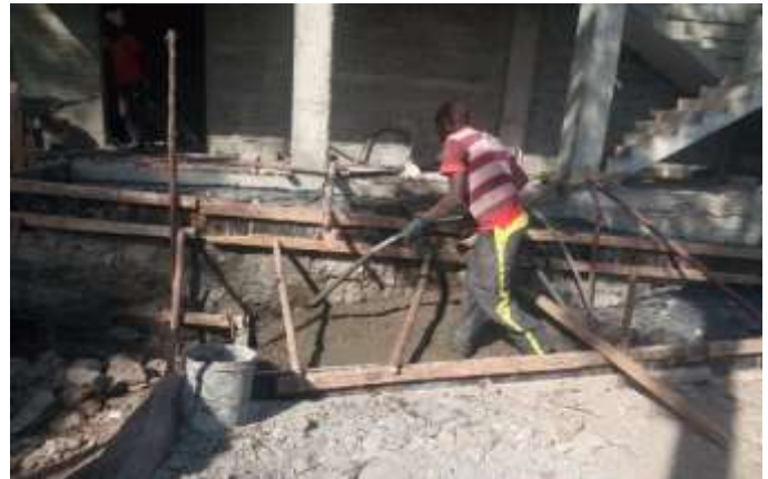
Ramp concreting
