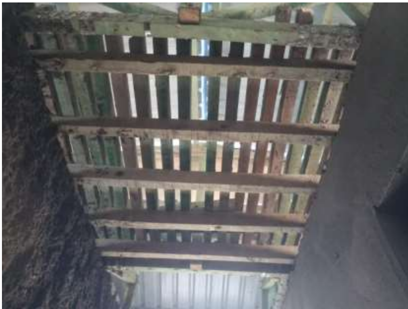
Platform for the water tank to carry 1,000 litres.
