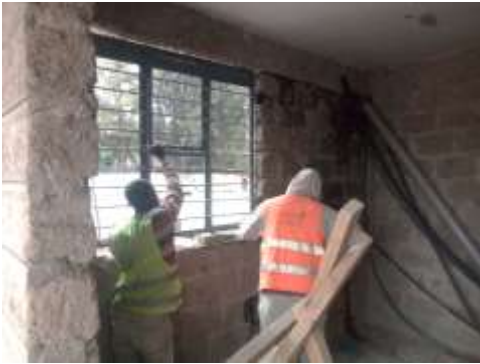
Fabricating and installing windows
