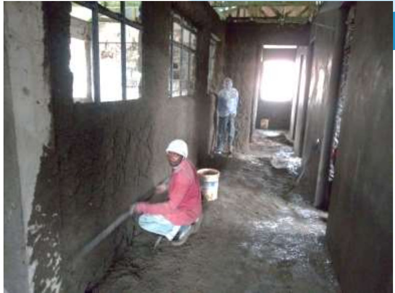
First floor plastering on-going
