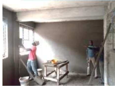
Ground Floor wall plastering
