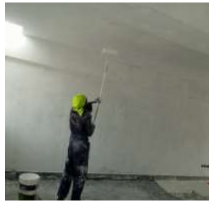
Under coat paint inside the classrooms.
