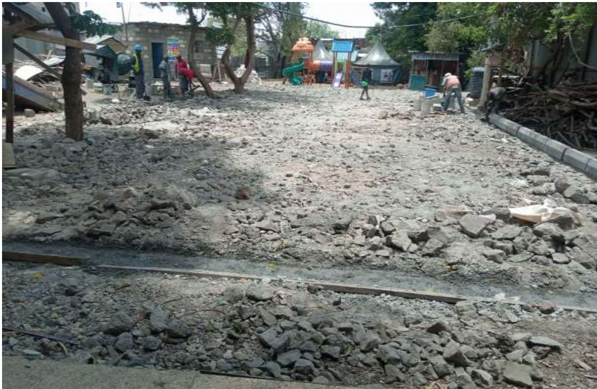
Leveling of the parking area
