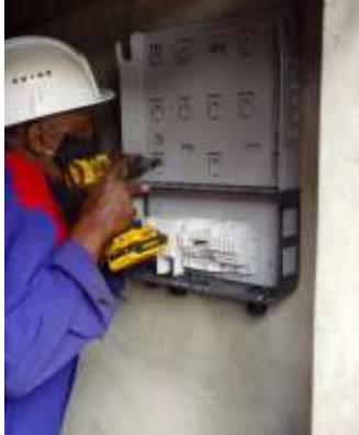
Installing Inverter box
