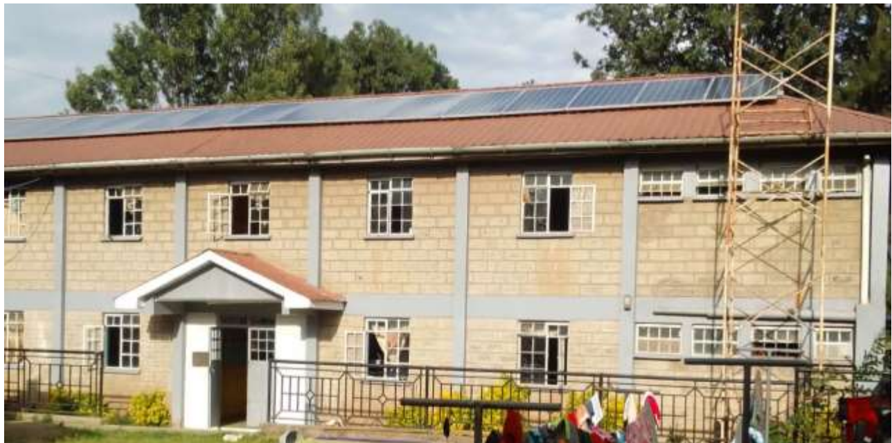
One side of the solar panels fixed.
