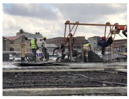
Steel works and Electrical conduits in place before the concrete pour.
