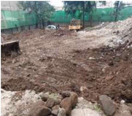
Clearing the site
