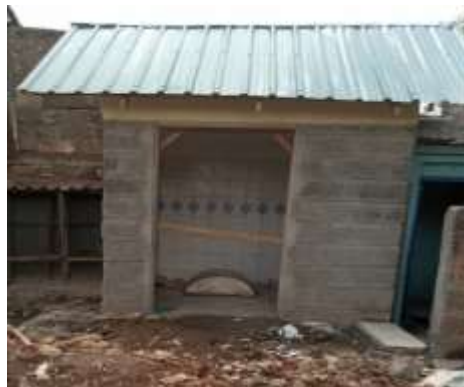
Disability friendly toilet nears completion
