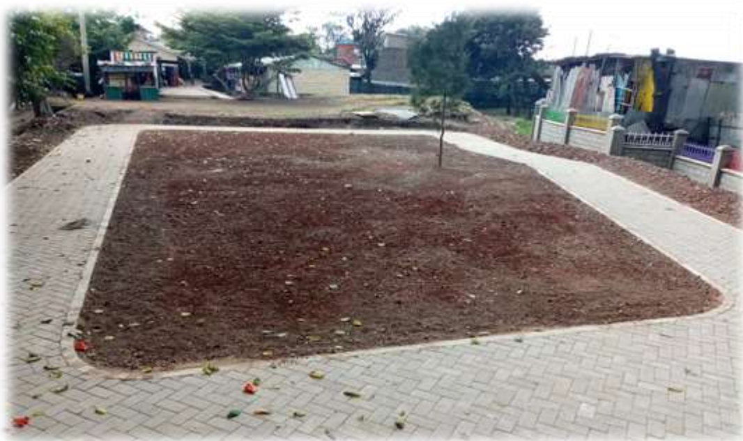
Levelled Ground and Wheelchair Circuit Completed
