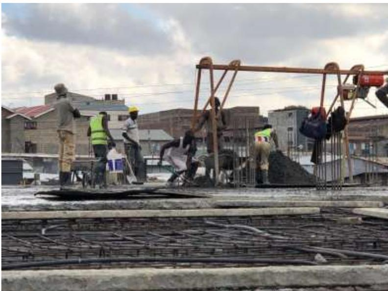
*Steel works and Electrical conduits in place before the concrete pour.*
