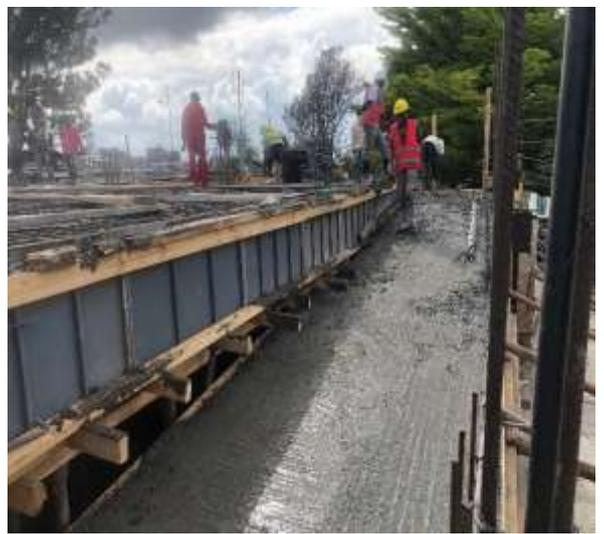
*End of September – Second Floor Slab concrete pouring and Ramp completed*
