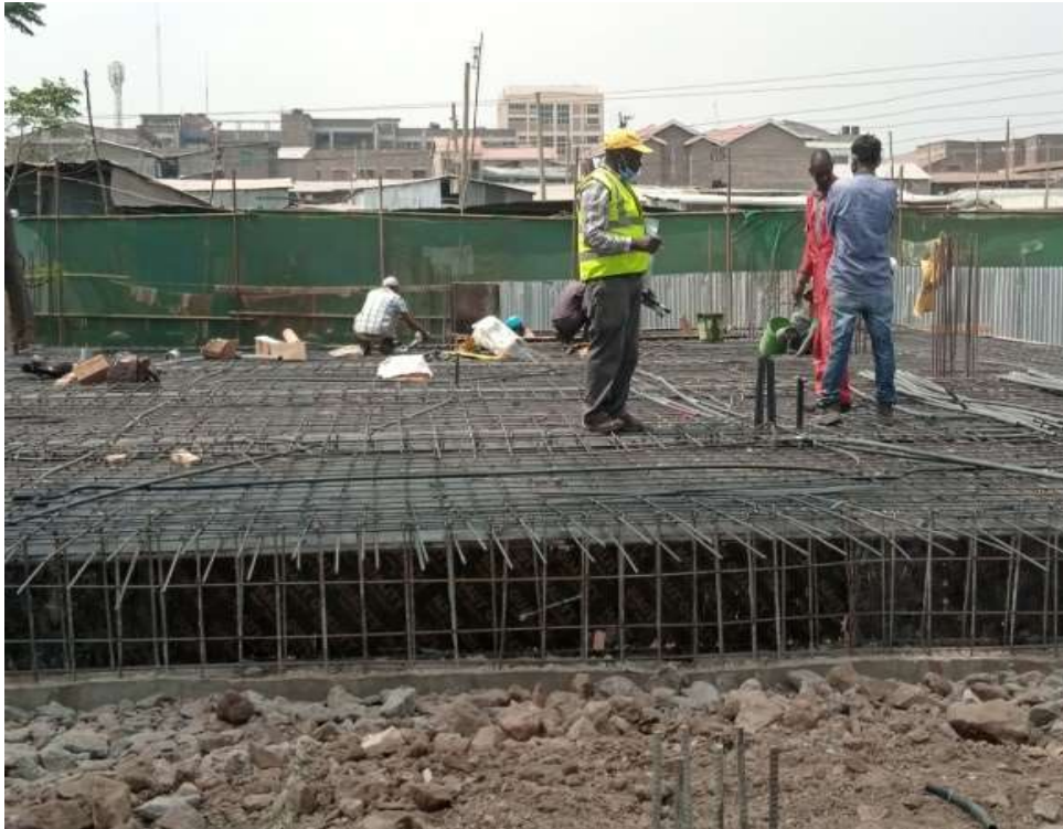
Electrical piping and steel fixing on the lower ground floor
