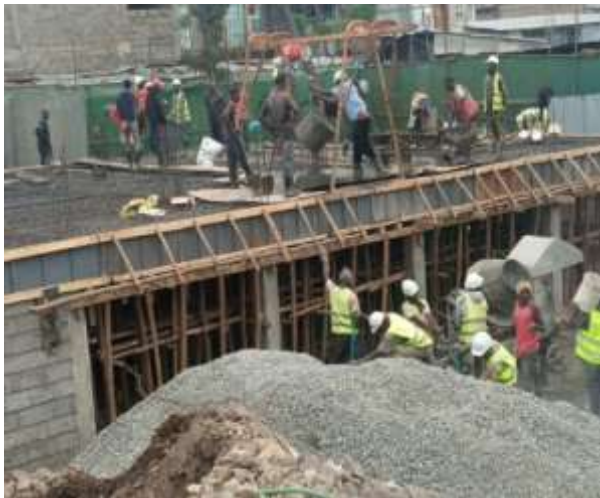
First slab work on the lower ground floor
