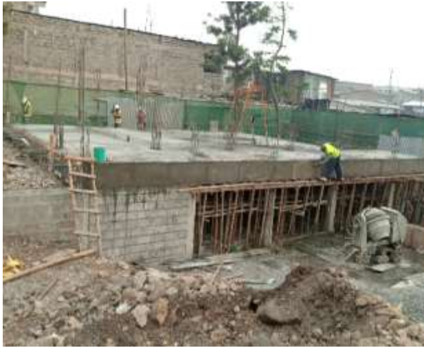
Concrete slab at the lower ground floor
